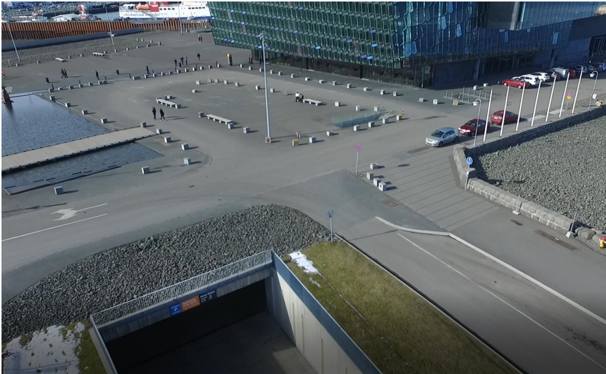
Figure 18 - Elevation from front of Harpa. Note concrete bollards, lack of marking, poor-visibility glass and badly-indicated water trench (ReSource)
