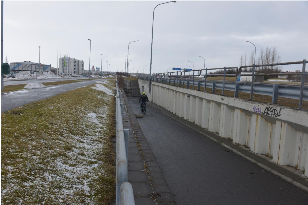
Figure 8 - Blind corner underpass at Mjódd, with long downhill slope encouraging acceleration and requiring braking (ReSource)
