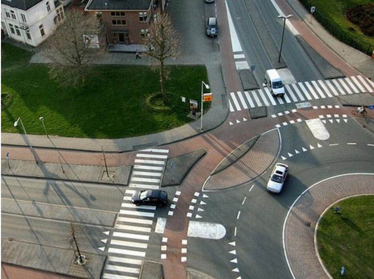
Figure 26 - Example of a convenient but dangerous design for cyclists, again from the Netherlands (source unknown). Lack of cycle awareness in Iceland is likely to make this design more dangerous.
