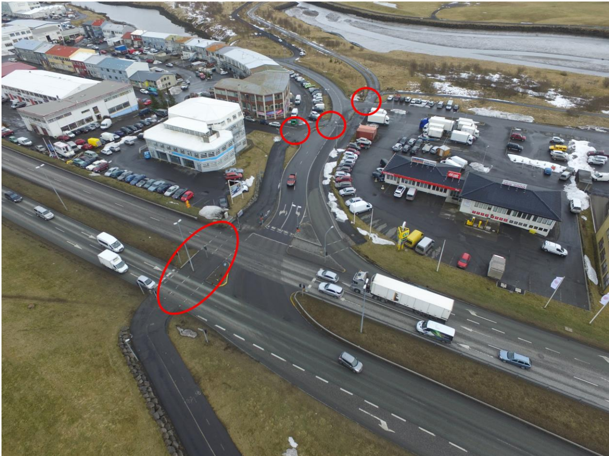
Figure 15 - Cycling junction at Sæbraut. Four road crossings can be seen. (ReSource)
