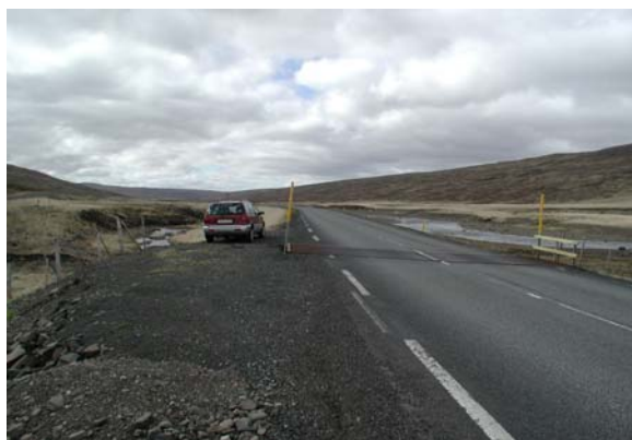
1 h3-05 Hringvegur, Fornihvammur
