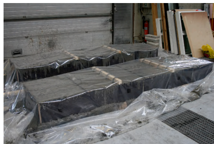
Figure 4-11. Beams wrapped with plastic after casting.
