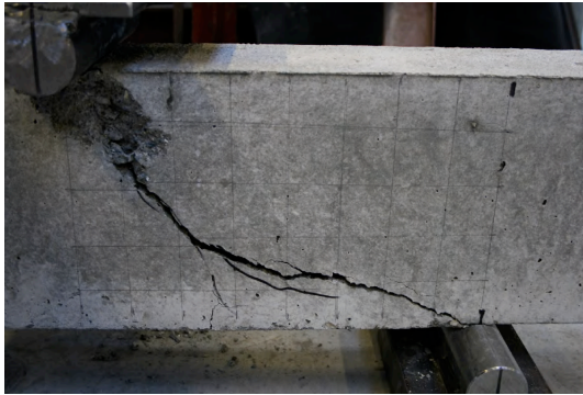
Figure 5-13. Crack pattern for BSb3 at ultimate load.
