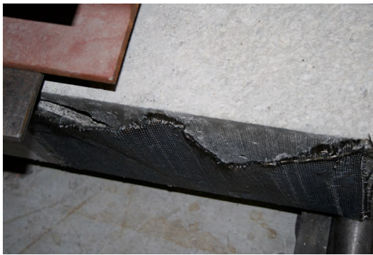
Figure 5-3. Bond failure, BSa3.
