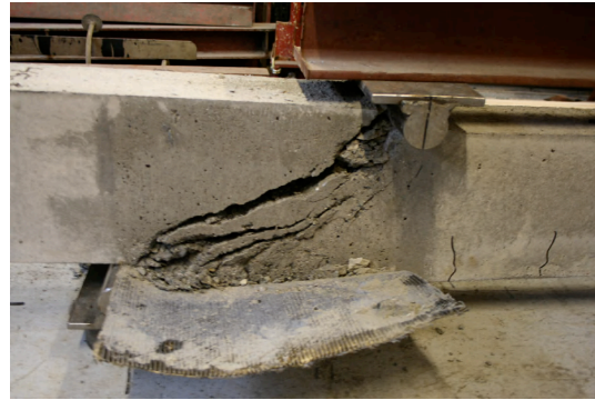
Figure 5-8. Crack pattern for BSa6 at ultimate load.
