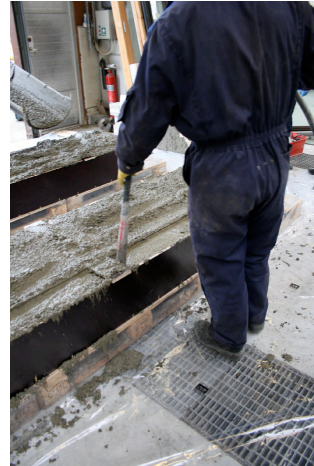
Figure 4-10. Beams vibrated.
