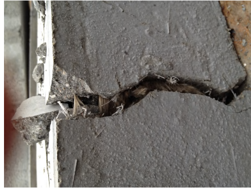
Figure 5-22. BFc5 (Fibre1), The fibres in BFRP sheet rupture.
