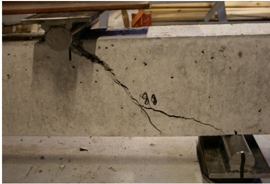
Figure 5-11. Crack pattern for BSb2 at ultimate load.
