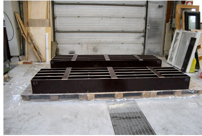
Figure 4-8. Formwork ready for casting.
