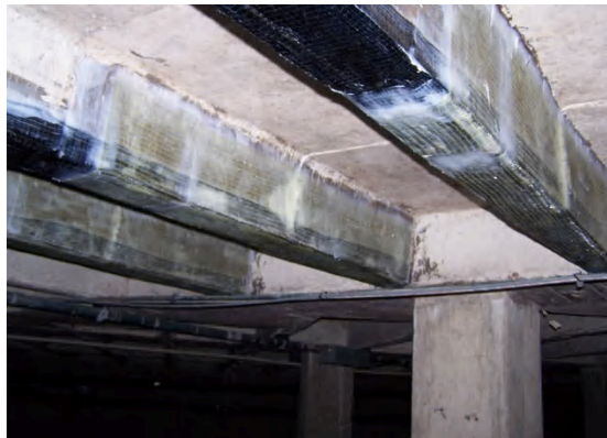
Figure 2-4. Shear and flexure strengthened beam [25].
