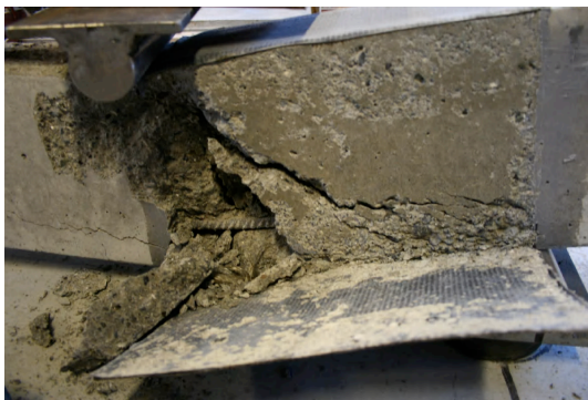
Figure 5-15. Crack pattern for BSb5 at ultimate load.
