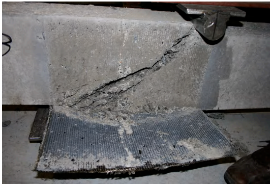
Figure 5-9. Crack pattern for BSa7 at ultimate load.
