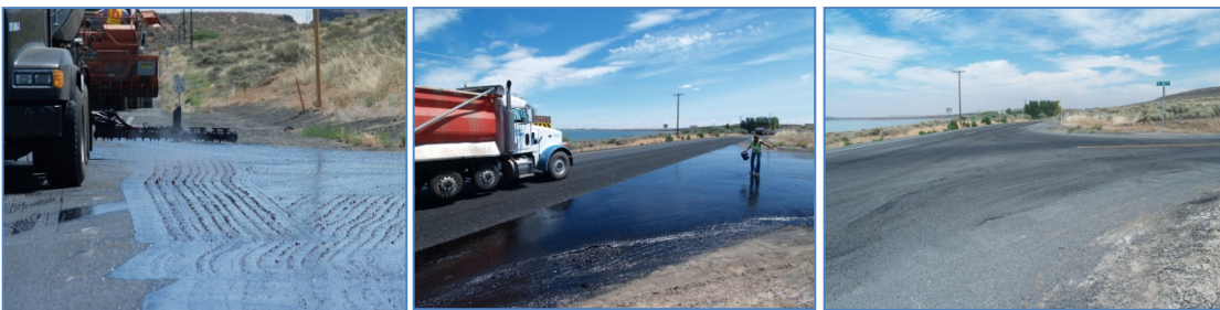
Figure 39 – Chip sealing an intersection
