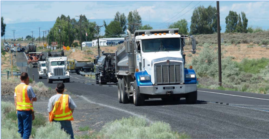
Figure 35 - Dump truck operators should try to drive on the non-wheelpath areas to ensure better orientation and embedment of chips in those areas.
