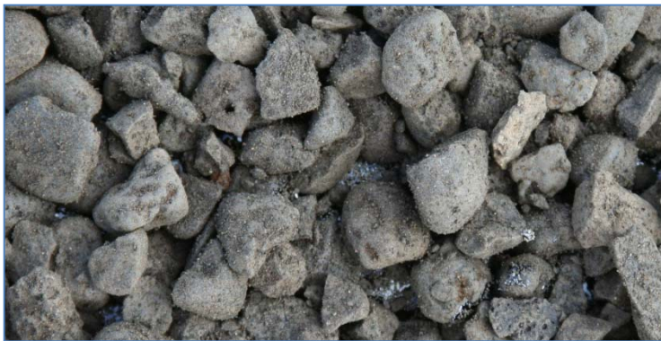
Figure 43 - Fairly round aggregate and insufficient embedment
