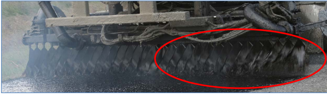
Figure 42 - The strong breeze is affecting the binder distribution
