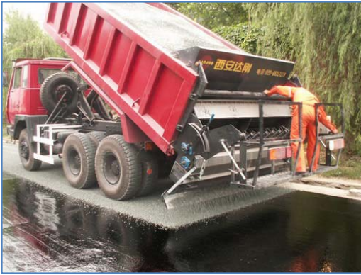
Figure 5 - dump truck box chip spreader.
