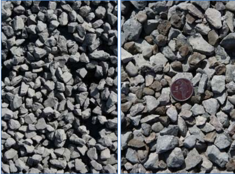
Figure 25 - First layer applied (left), second layer, choke stone applied (right)
