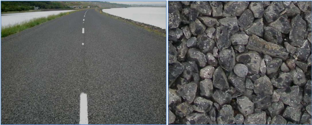
Figure 30 - Eyjafjordur finished surface
