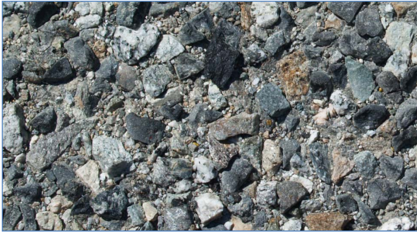
Figure 22 - choke stone chips fills up the voids between the larger chips
