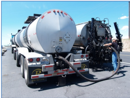
Figure 2 - Asphalt hauling tank filling up a binder distributor tank.
