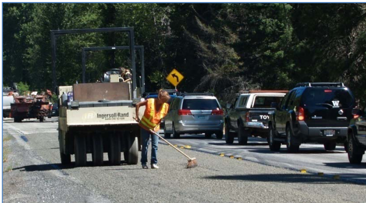
Figure 8 - Roller operator covering a bleeding wheelpath before rolling
