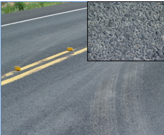
Figure 32 - Existing BST pavement was in good condition
