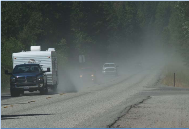
Figure 17 - Result of a dusty choke stone.
