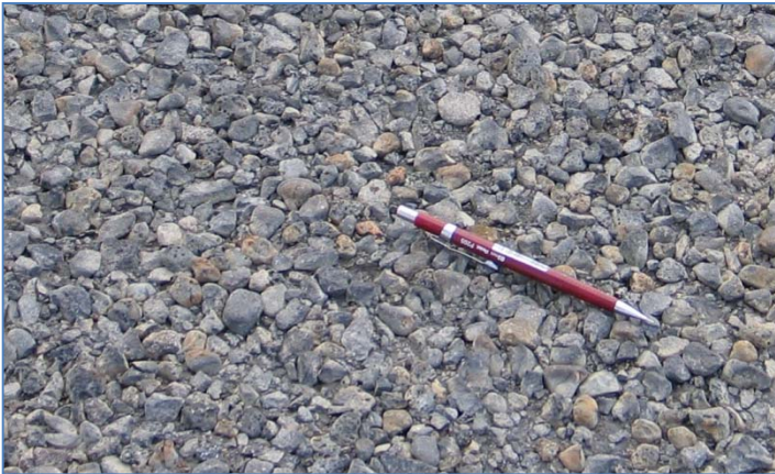
Figure 47 – Gaulverjabaer R 829 finished surface
